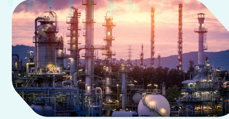
Petrokimya ve Rafineri Petrochemical & Refinery Industry
